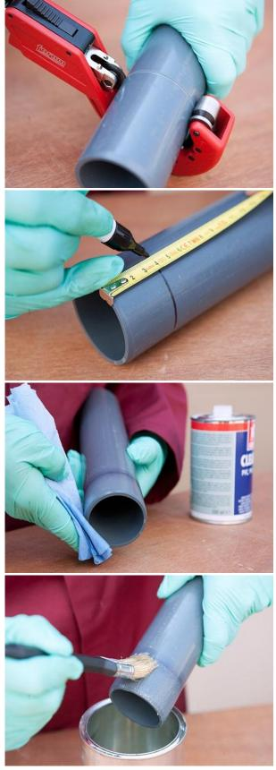
Cut the pipe end squarely, remove internal burrs and chamfer to 15°.
