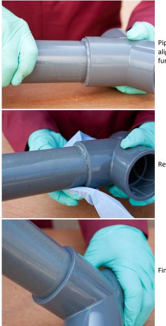
Pipe and fitting should be joined slowly and in correct alignment & restrained. 15min waiting time before further cementing below 10°C wait 30 min.
