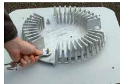
Unscrew the nuts and lift the leafguard grid to remove it.
