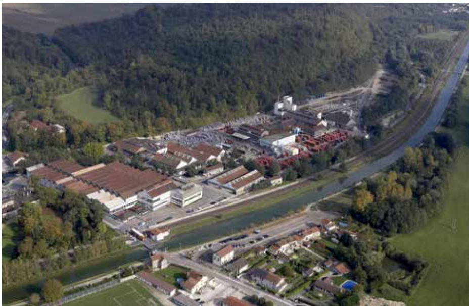
Bayard plant (Haute-Marne): ISO 9001 and ISO 14001 certified by Bureau Veritas.
