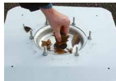
Clean the inside of the roof outlet bowl.
