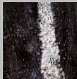
Zinc coated: a white line of zinc salt shows that the damage is completely plugged
