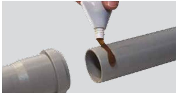
When inserting, the ring seal must be free of lubricant. Center up the spigot end of the pipe and push until the pipe end reaches the end of the socket.
