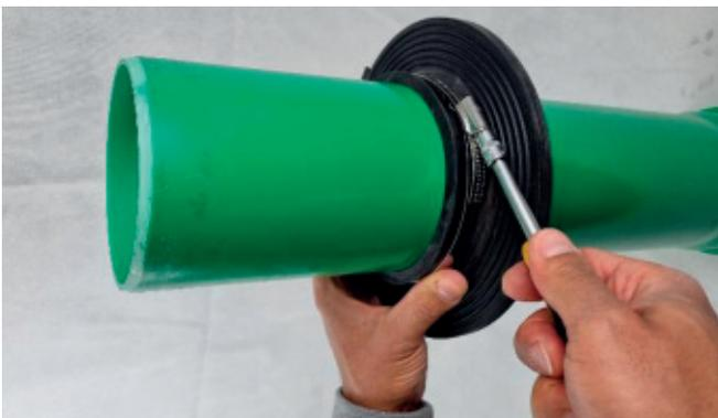
Fasten steel straps on both sides around the wall collar.
