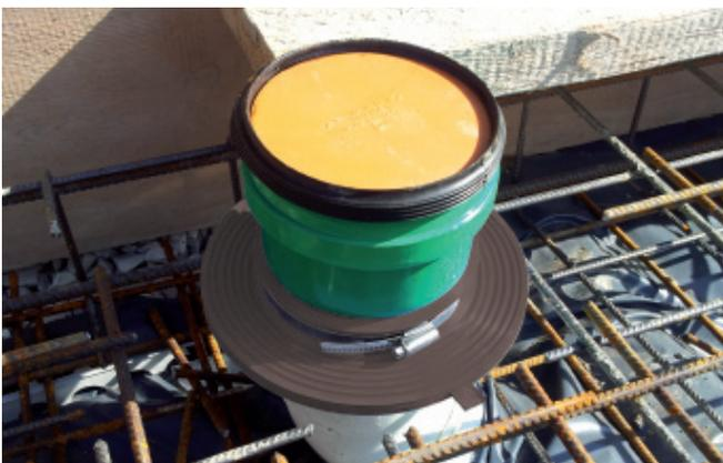
The 4 pipes wall collar is now ready for casting in core hole or wall sleeve.
