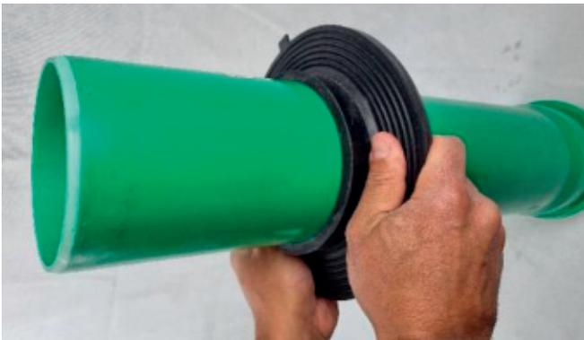
Put wall collar on the medium pipe and center the position of wall sleeve ore core hole.
