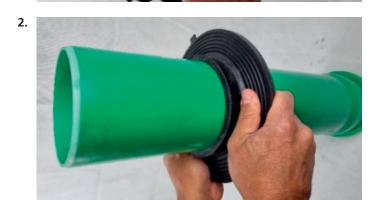
Put wall collar on the medium pipe and center the position of wall sleeve ore core hole.
