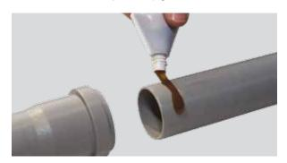
When inserting, the ring seal must be free of lubricant-Center up the spigot end of the pipe and push until the pipe end reaches the end of the socket.
