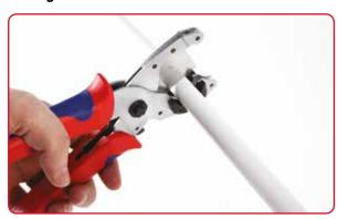
Use a set of Maincor Cutters to enable a straight and accurate 90° cut on the pipe.
