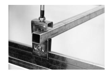
7. Slide A centre bracket onto the square bar, mount the outlet reducer through the A centre bracket and lightly tighten the nut. Adjust location of the centre bracket and the side B brackets until desired location of the outlet reducer is achieved. Firmly secure the side B brackets by tightening the screws to a torque of 5 Nm/4 ft-lbs.
