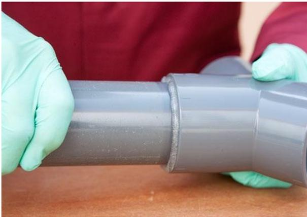
Pipe and fitting should be joined slowly and in correct alignment & restrained. 15min waiting time before further cementing below 10°C wait 30 min.
