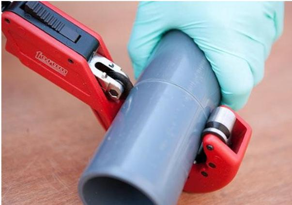
Cut the pipe end squarely, remove internal burrs and chamfer to 15°.
