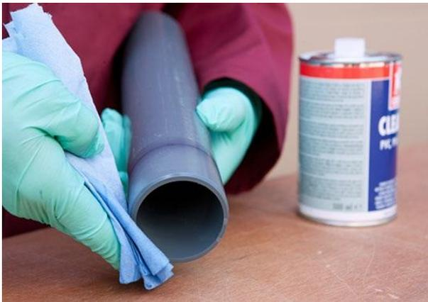
Clean pipe and fitting socket thoroughly with PVC-U cleaner.
