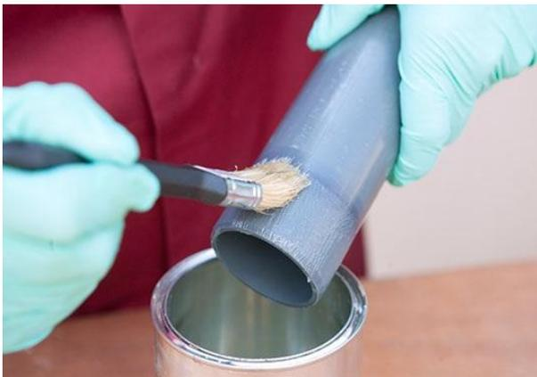
Apply solvent cement in the middle of the pipe cementing surface & distribute it first radially than axially all over.
